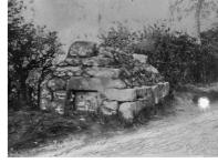
Lands of Fountainhall, erected in connection with the first city water supply 1706, Re-erected 1903'. Rectangular pool in front, with four stone steps on each side leading down to water; brick and stone lined vaulted inner chamber. Moved from near Fountainhall House, now 130 Blenheim Place, as shown in the above photo.
