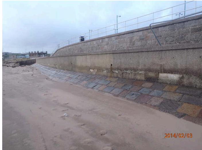
The third part is made up of two walls and a poured concrete footway which has some sand covering it. The wall nearest to the sea presents vertical cracks and carbonation in the down part of the wall.
