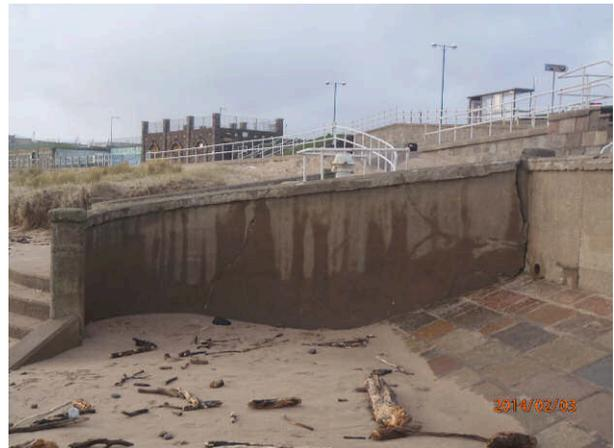
The other stairs is in very bad condition because it has lost the last two steps completely, for that reason have been closed with fence but the water and wind have moved it.
