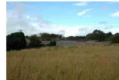
Viewpoint 17: Electricity Substation
