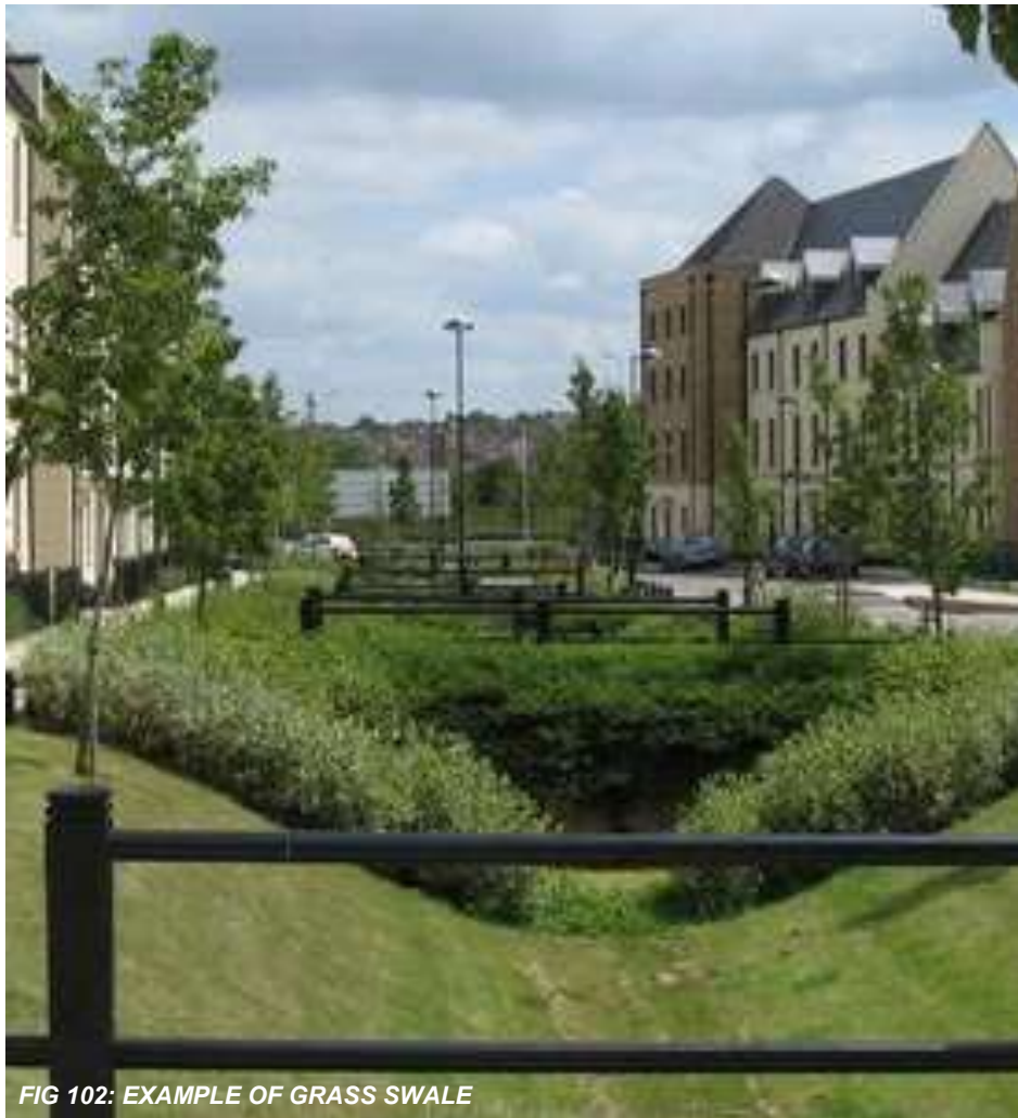
FIG 101: EXAMPLE OF GRASS SWALE
