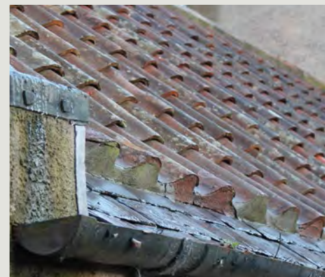
Figure 5.57: Traditional eave detail
