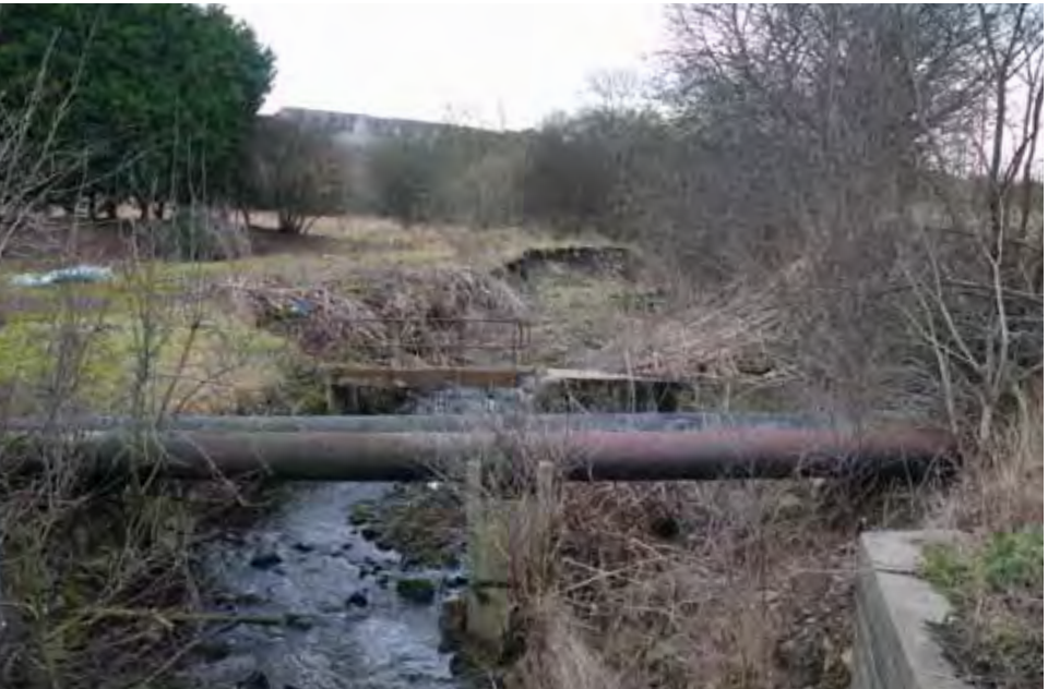
Remove redundant grilles, pipes and infrastructure
