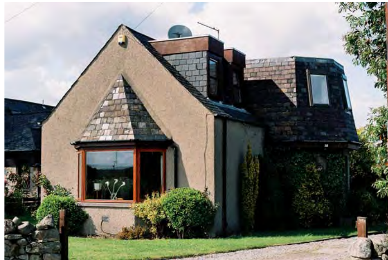
Urban style dormer windows (and bay) on a residential steading conversion. Apart from the gable end the adaptation leaves very little to express the building's original function.
