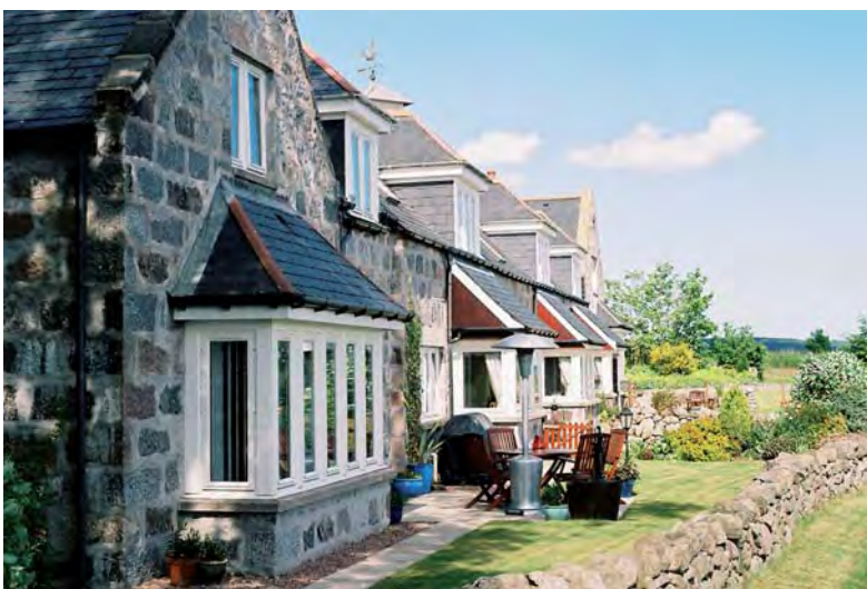
A residential steading conversion to several units using high quality materials and appropriate boundary treatment, but with an accumulation of new window openings of a domestic scale and style. These new openings conceal the original simple character of the building.
