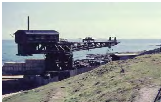
Titan crane at the Breakwater.
