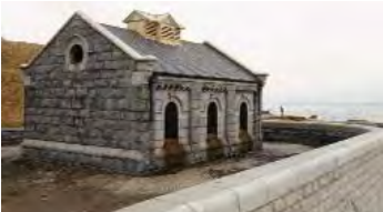
Sewage Valve House.
